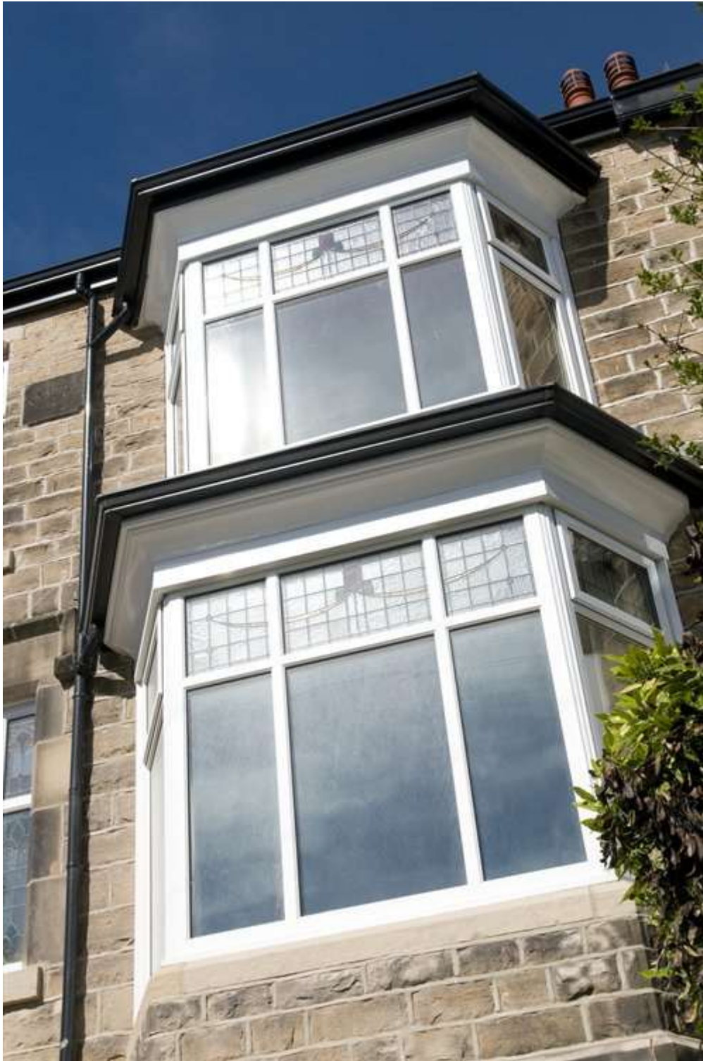
uPVC Bay window installed in a traditional stone property
