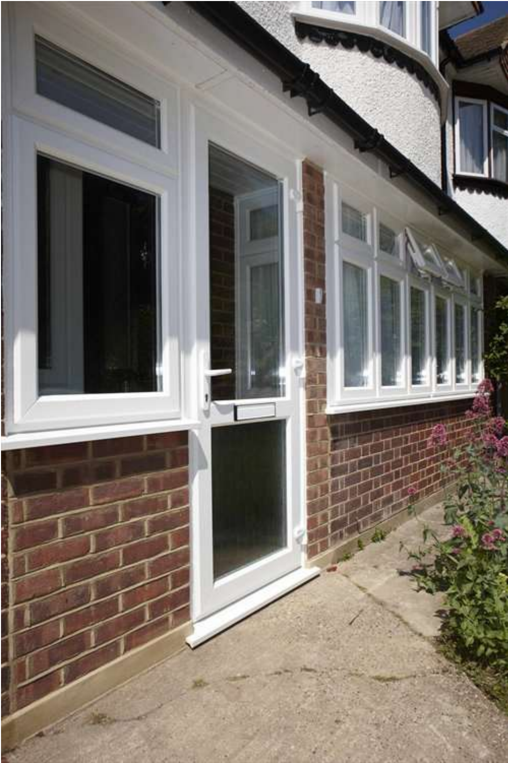
Double glazed Entrance Door
