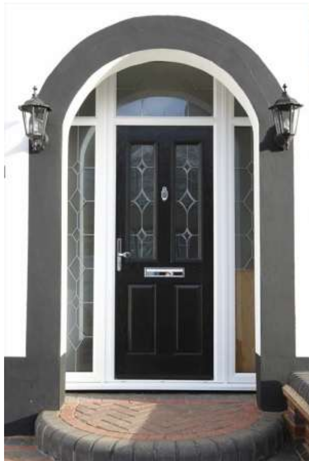
Entrance Door with Side Lights
