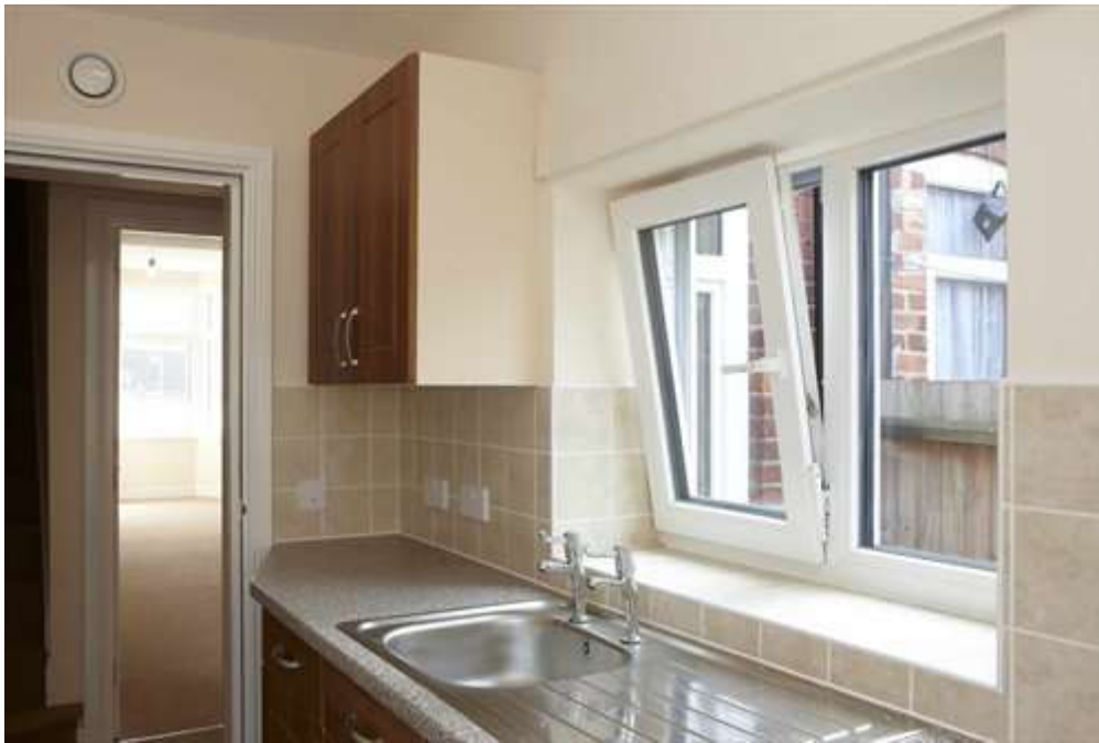
uPVC Tilt & Turn Window – Tilt Position
